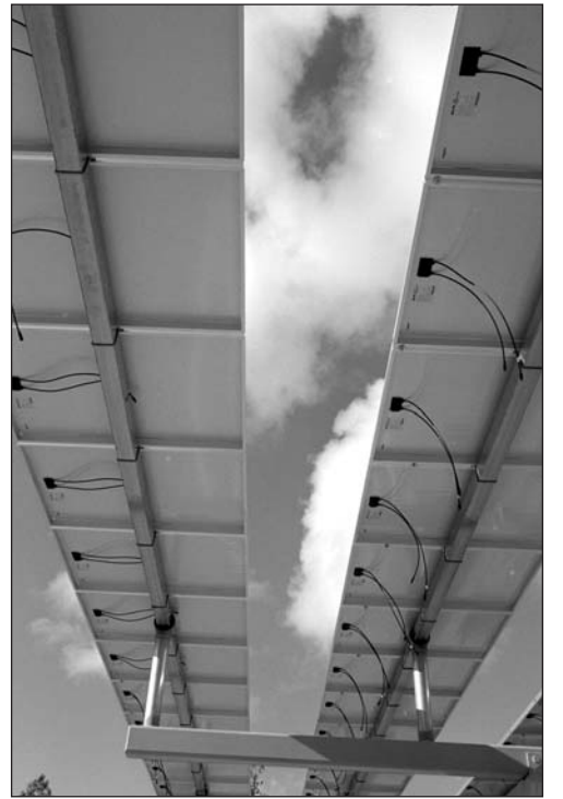
Left: Solar panels sits on top of the Lot C parking structure. Bottom: The solar panels are controlled by two motors following the sun's movement.
