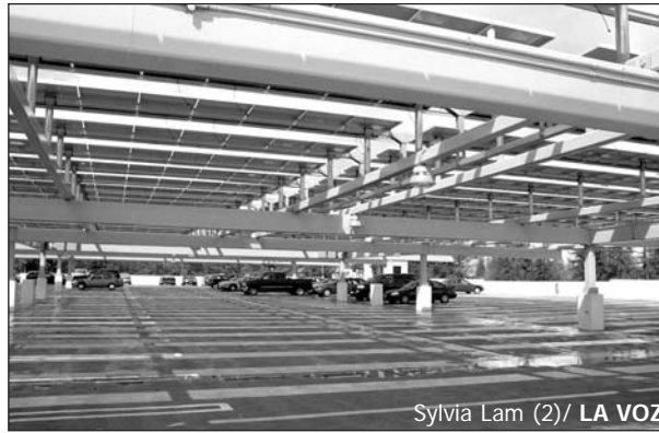
Left: Solar panels sits on top of the Lot C parking structure. Bottom: The solar panels are controlled by two motors following the sun's movement.
