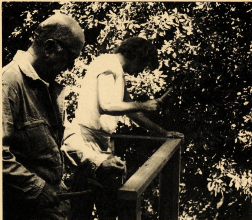
Maxwell (right) puts finishing touch on railing.
