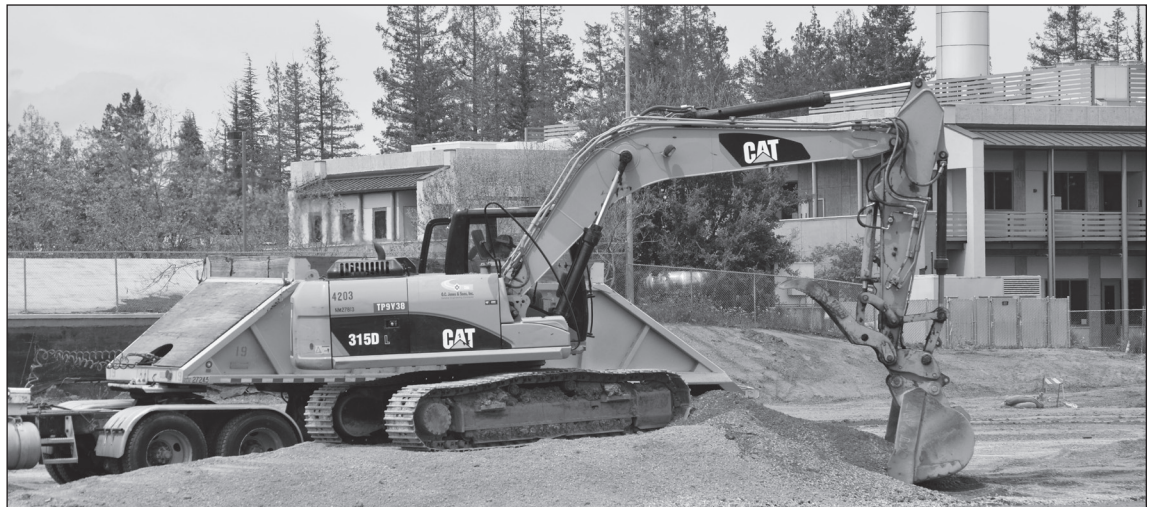
Heavy Equipment - Construction workers remove a pile of dirt from where the old field used to sit. A new, NCAA rated track and field will be installed and is expected to open late in fall quarter 2012.
