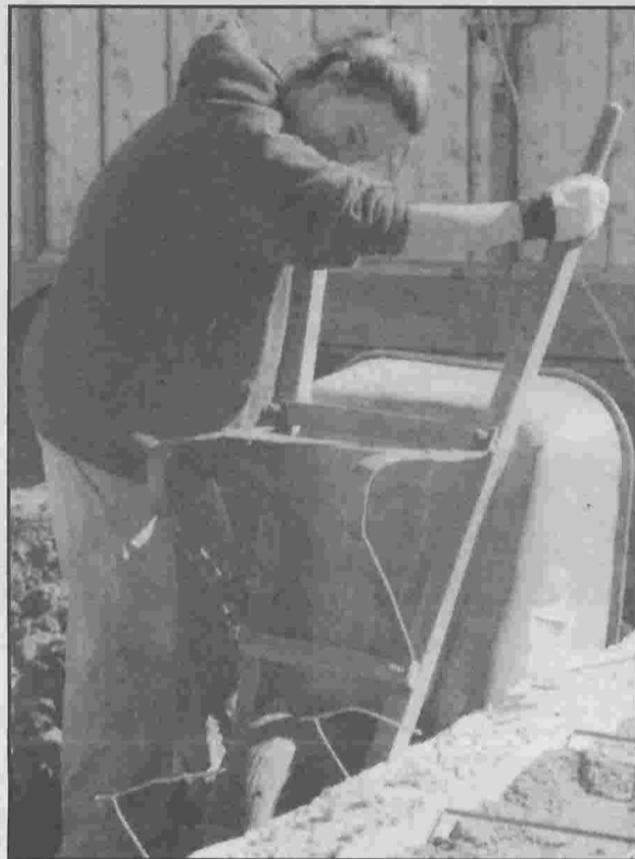
The students who will build and renovate homes over spring break are being trained in tiling, dry walling and door hanging by Home Depot. This and other businesses are donating time and supplies for the City Year project.
