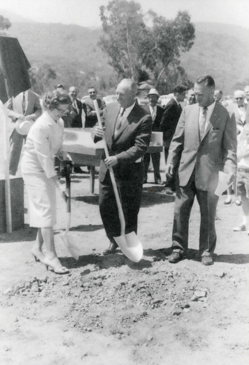
Mary S. Levine, A.P. "Pete" Christiansen, and Cal Flint break ground for the permanent Foothill campus.
