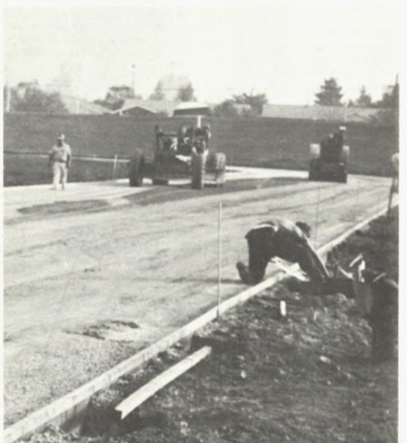
The De Anza track, still under construction, will be the best in Northern California, according to track coach Don Vick. (La Voz photo by Dennis Bellman)
