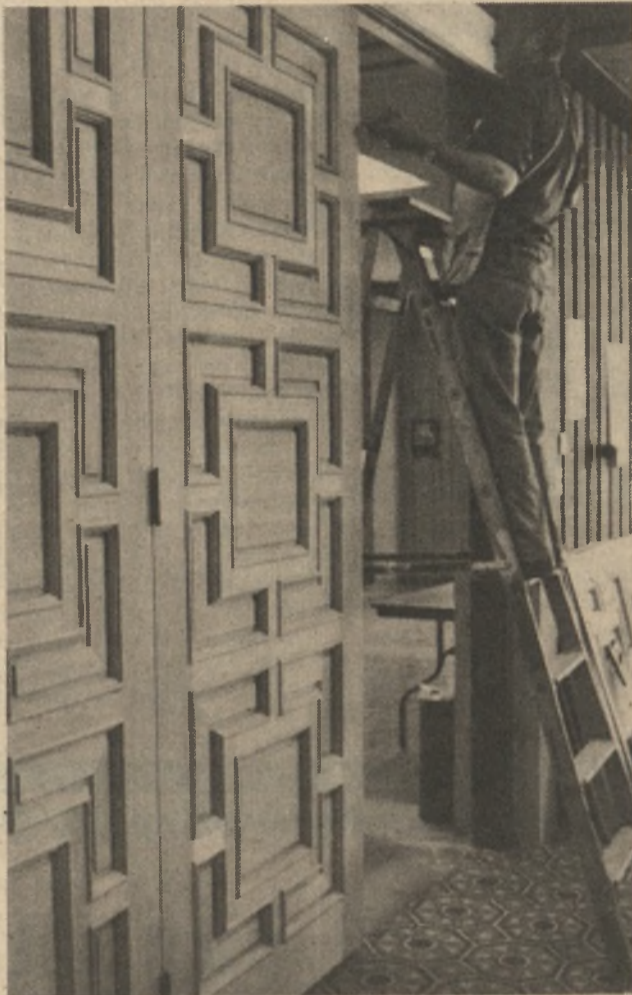
Photo by Marcia Edelsten Steve Blake of Stavv Construction Co. Palo Alto, installs the three Philippine mahogany doors on the Campus Center El Camino Room. The doors were made in Mexico to match those hung on the main dining room in 1970.
