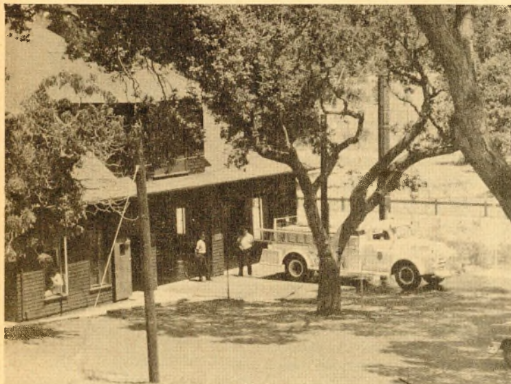
THIS IS exterior view of the building housing Foothill's fire protection—as well as that of Los Altos Hills. It's the Foothill substation of Los Altos Fire Department on campus, opened May 1. Story and more pictures on page 4.
