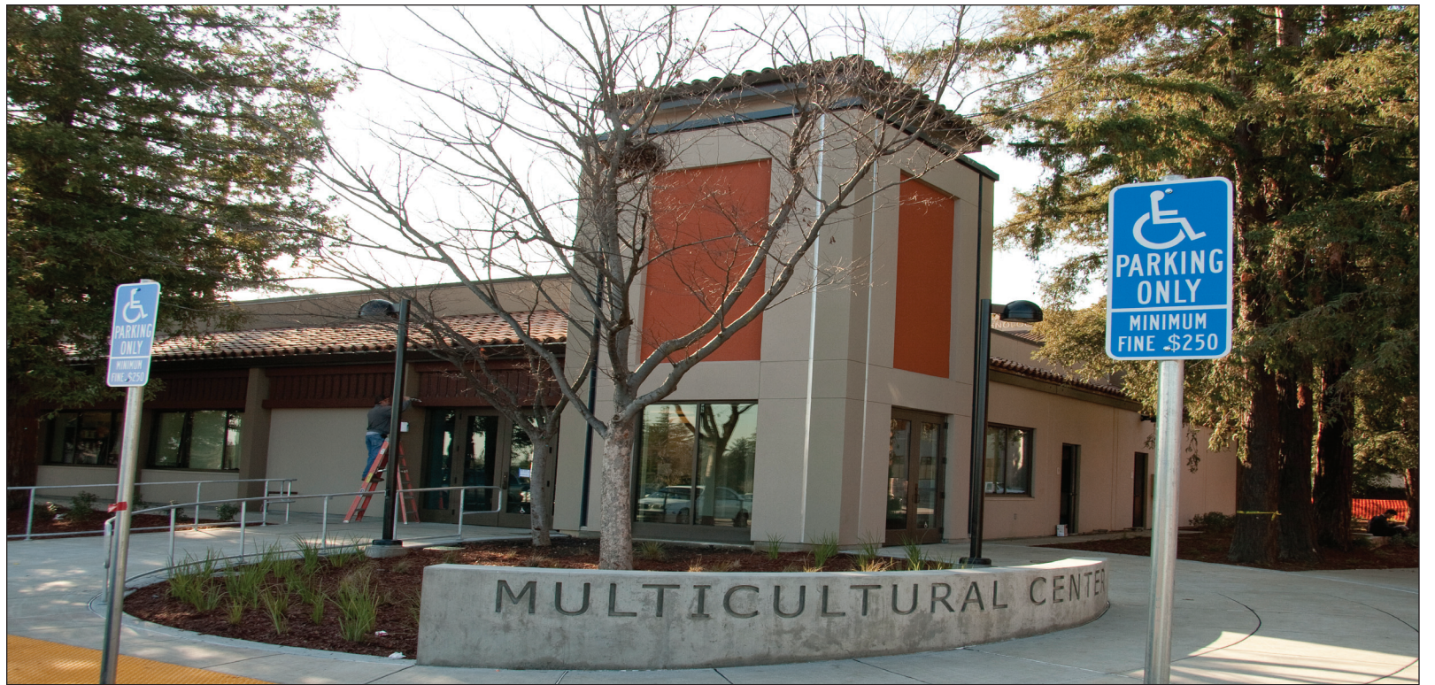
FINISHING TOUCHES - Construction workers make final details on the retrofitted Multicultural Center, giving polish to De Anza College's latest building opening.
