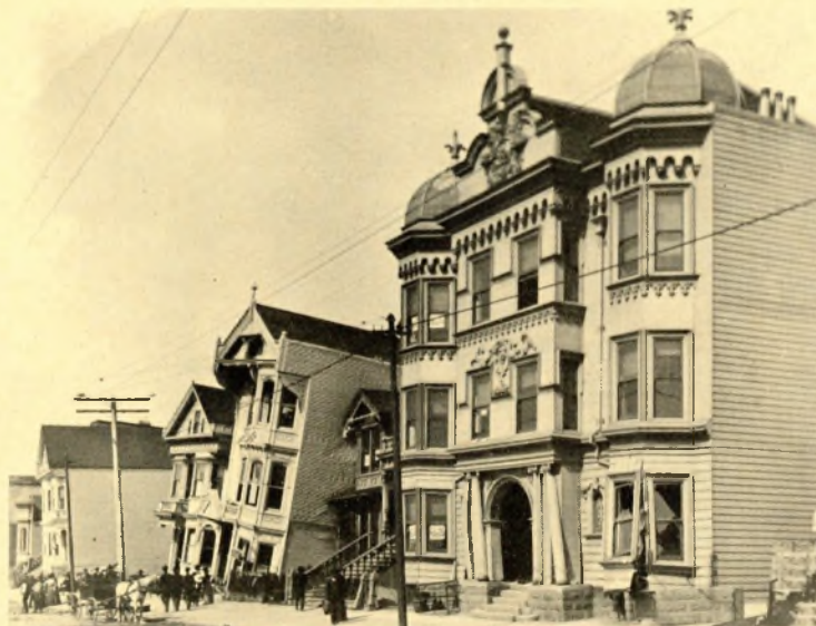
The San Francisco quake toppled these houses on Howard Street in the Mission district. This section of town was built over loose fill.*
