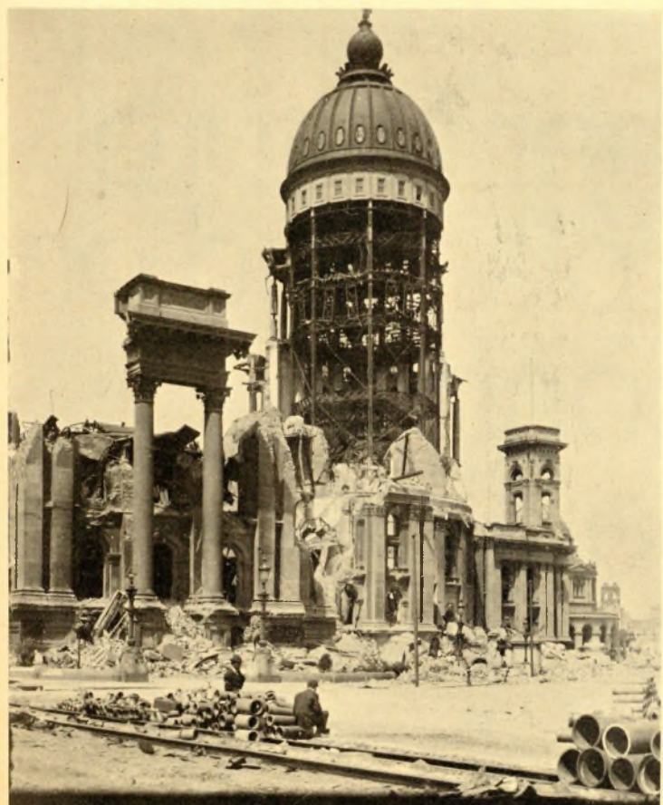
The shock of the 1906 quake stripped the stone and marble sheathing San Francisco's recently completed $7 million city hall and left the steel construction standing.*
