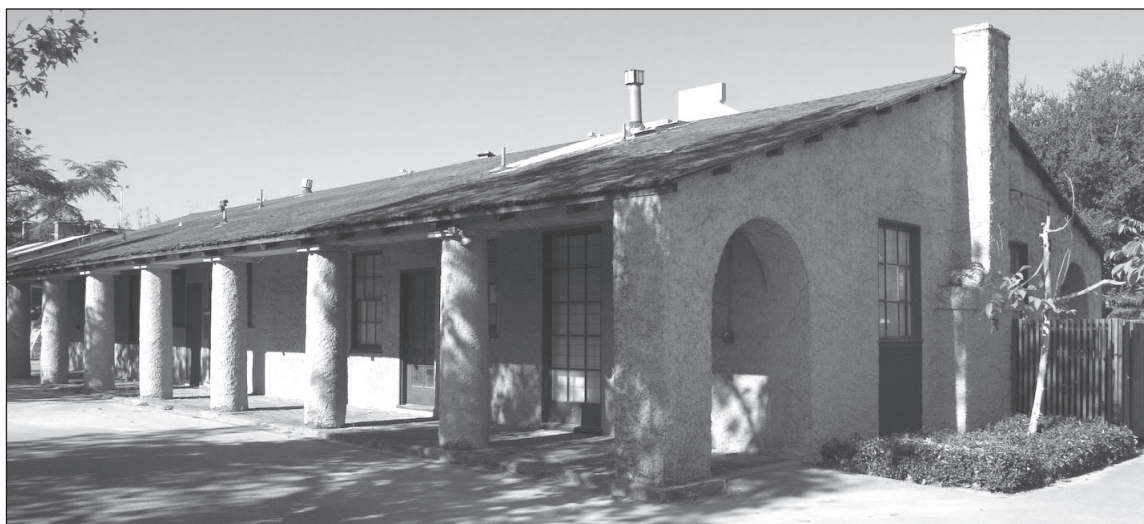
Some the architectural elements found in the cottages are stucco walls, long corridors, tiered arches and curved gables. The original designs influenced on other De Anza College buildings, such as the Hinson Campus Center and the new Student and Community Services Building.
