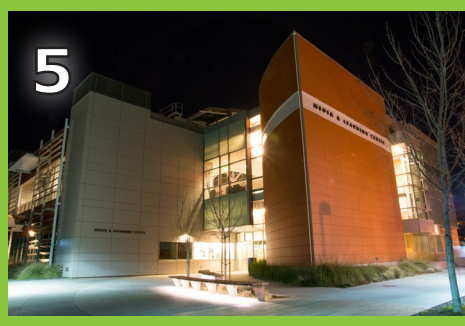
5 Media and Learning Center • Rooftop solar panels for both electricity generation & heating water • Advanced energy efficient ventilation system • Windows and skylights designed to let in maximum daylight • Orientation and layout for maximum energy efficiency • Water conservation controls including drought tolerant landscaping • Radiant heating in the lobby/atrium floor
