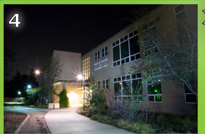
4 Kirsch Center for Environmental Studies • The first community college Green Building nationwide to be certified LEED Platinum • Home to the Biological, Health and Environmental Studies • Home to the Cheeseman Environmental Studies Area • Rooftop solar panels for both electricity generation & heating water • Advanced natural ventilation & radiant heating and cooling • Orientation and layout for energy efficiency and passive solar benefits • Water conservation controls including drought tolerant landscaping
