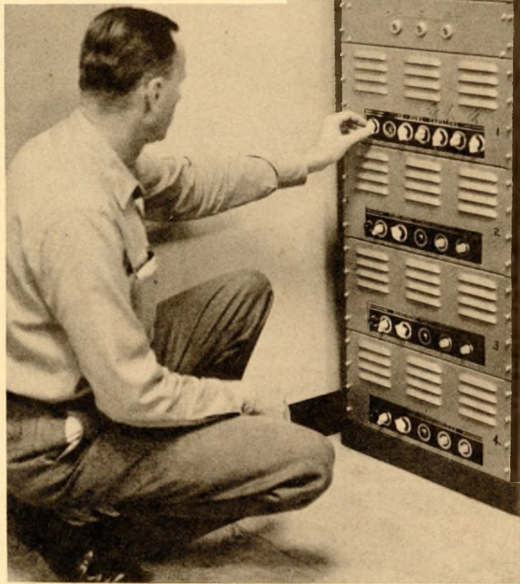
FIX-IT MAN —George Bruns is shown tuning the chimes that are a distinctive Foothill feature. Bruns is also responsible for the maintenance of many other mechanical and electrical systems on the campus.
