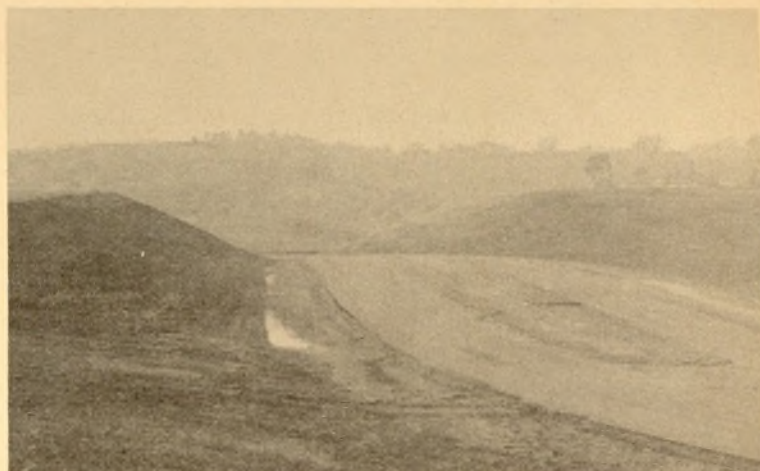
TODAY BECOMES TOMORROW—After the graders came the rollers, and soon the main entrance road bed was finished. I could hardly believe my eyes when I saw the architect's model of the same area in 1961.
