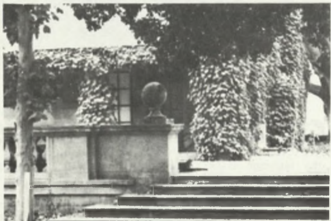
The guest cottages from the old Euphrat estate are now being used as guest faculty offices. The future fate of the structures is still undetermined. (La Voz photo by John Jean)
