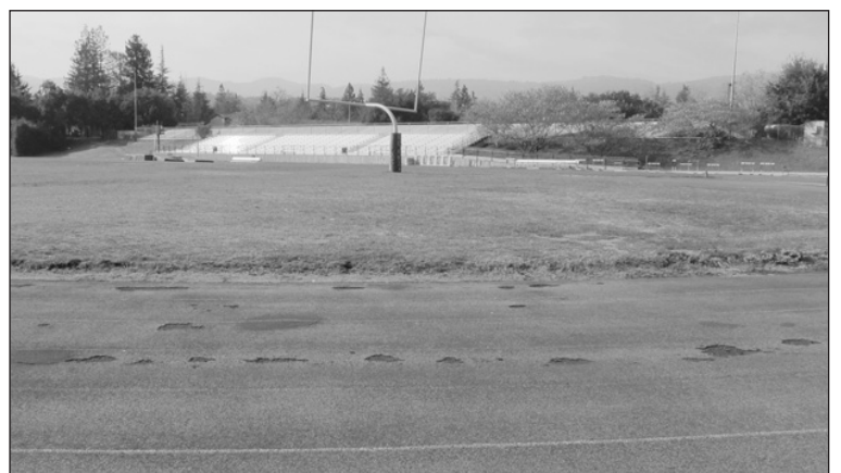
POCKMARKED - The north end turn of De Anza's current track is marked with holes.
