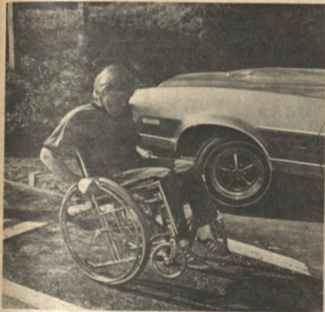
Newly constructed ramps aid DAC handicapped.
